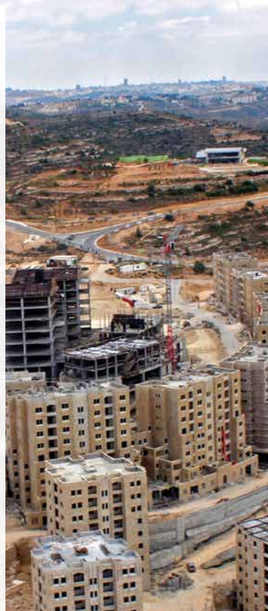
THIS PAGE: Construction is underway on Palestine's first planned city, Rawabi.
